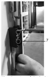
The direction of the lock is changed. Screws are assembled as shown.
