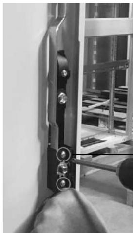
The lock is removed by unscrewing the 2 screws shown above.
