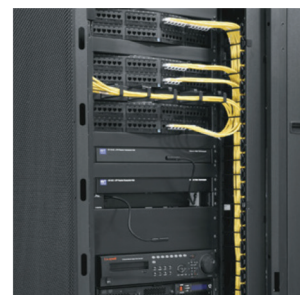
Internal Cable Duct
