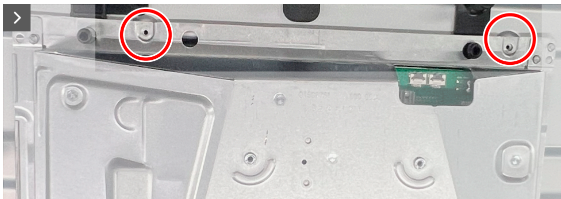
Figure 22. Removing the metal shield
